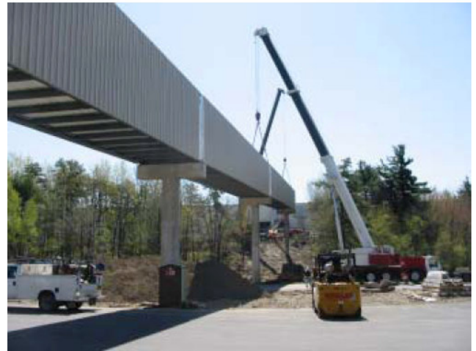
Looking from the packaging firm to the client's facility
