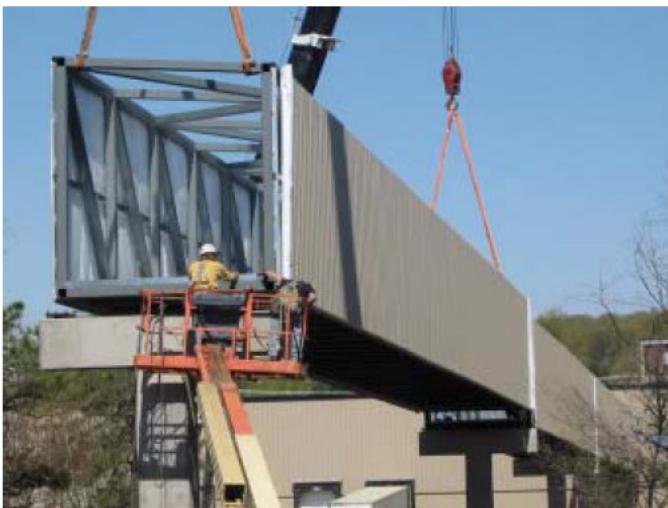
Setting bridge section on bearing plates
